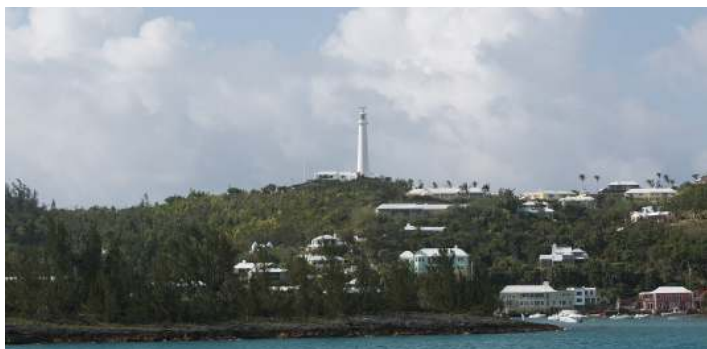
Gibbs Hill Lighthouse above Southampton Parish
