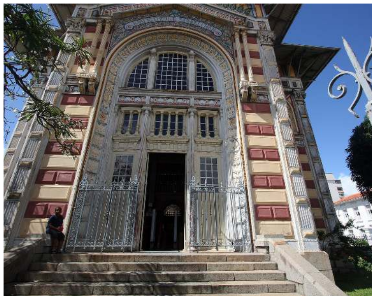
The Schoelcher Library, Fort-de-France
