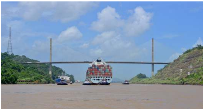
The Culebra Cut and the Centennial Bridge
