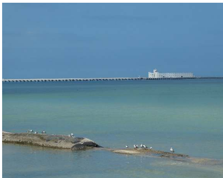
The causeway pier running out to the cruise berth
